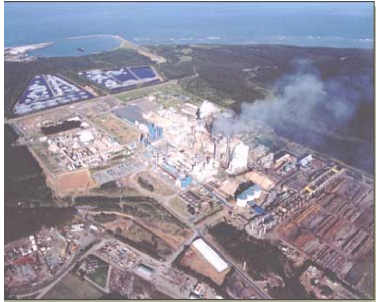
Aracruz Celulose bleached eucalypt kraft pulp mill in Barra do Riacho, Espírito Santo, Brazil Largest in the world
